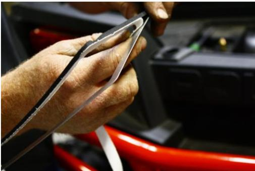
**Step 5:** Attach a foam gasket to each side of aluminum plate. **(as seen to the left)**
